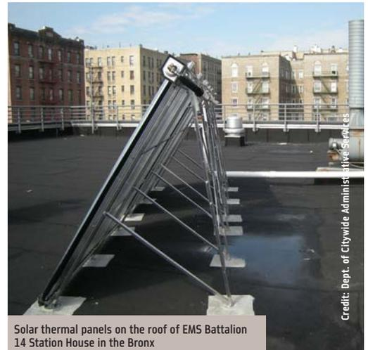
Solar thermal panels on the roof of EMS Battalion 14 Station House in the Bronx
